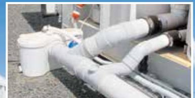
Fixtures from a complete bathroom are drained into the Sanibest Pro.
