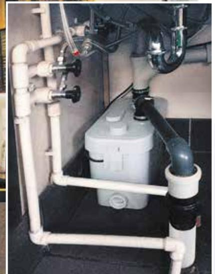
Sanivite installed underneath the counter sink
